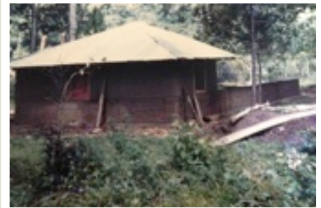
Construction of the Blumenschein Clinic
