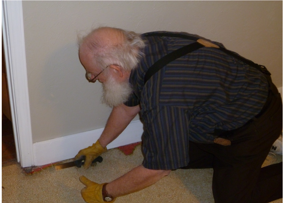
After moving into the Luff Home in January, Charlie Robison removed worn-out carpet.
