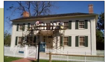
Mansion House gets repairs.
