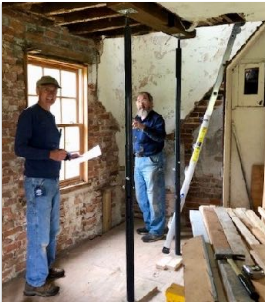
Volunteers do restoration work on the Clark house in Nauvoo.
